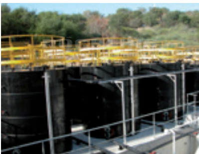
Polystone® G black B 100-RC 盐酸储液罐
